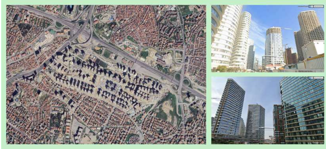
Figure 2. Images from the project area, which is high and not in harmony with its surroundings (Google Earth, 2025).
